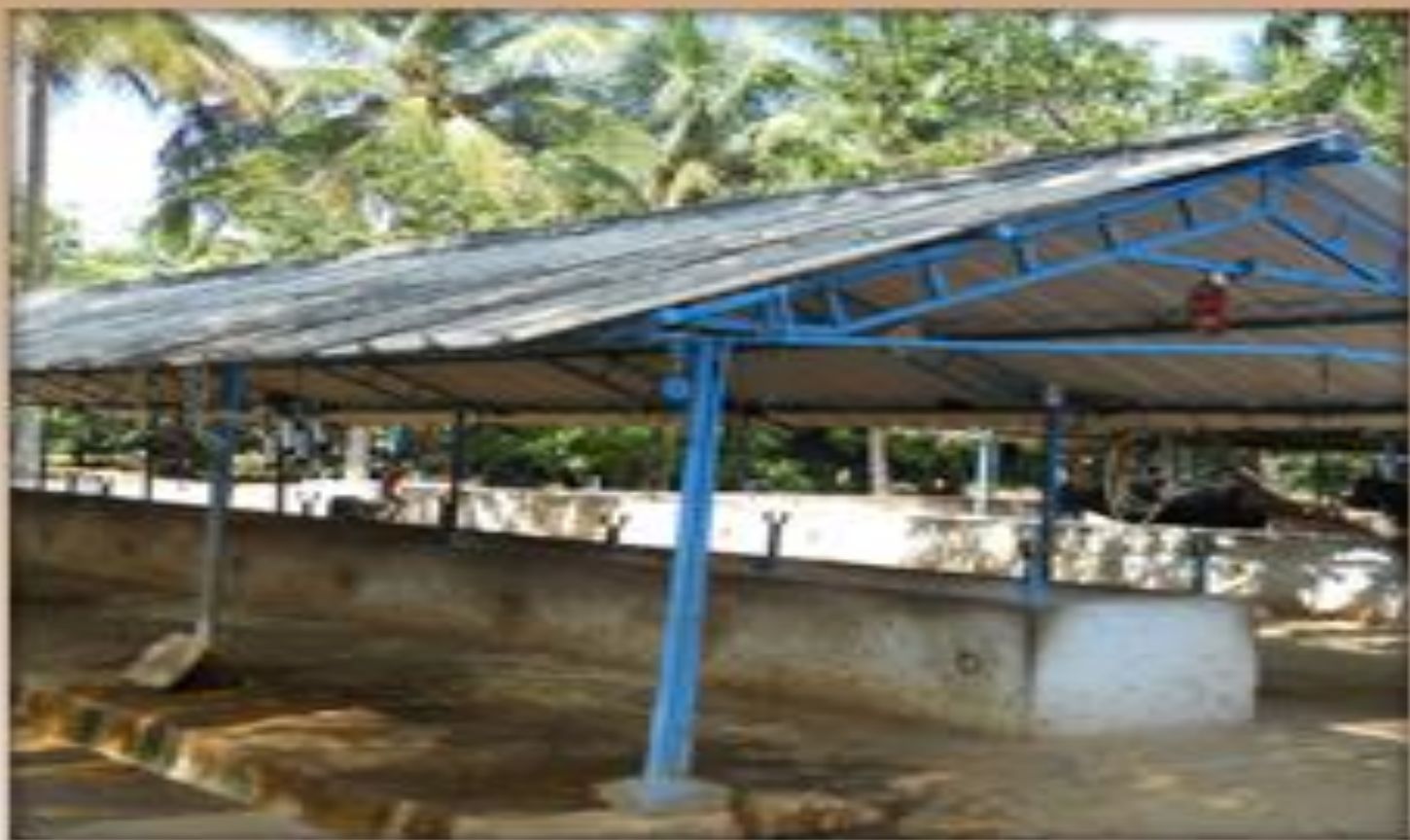
Asbestos Sheet Roofing
