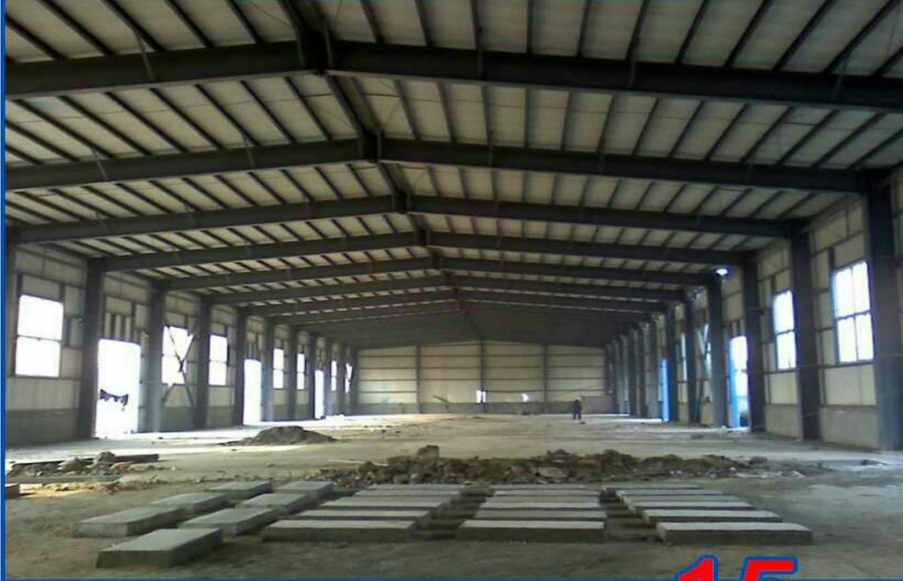
Galvenised iron sheet roofing
